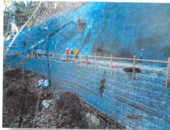
MSE Wall – Flume 51 Replacement
