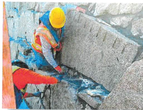
Grouting Stacked Rock - NCPA Union Dam
