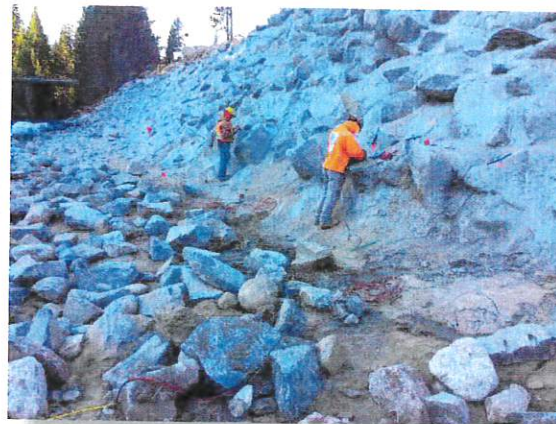
RSP - Eastwood Visitors Center Bank Stabilization
