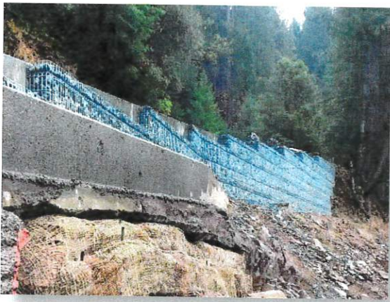
MSE Wall – Brush Creek Boat Ramp
