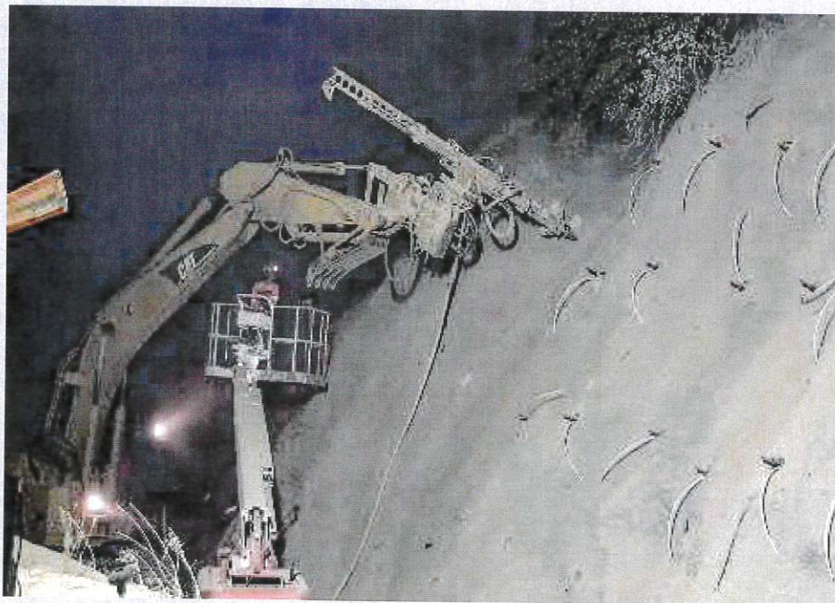
Figure 7 depicts an excavator mounted drill on a recent SMCI Job.
