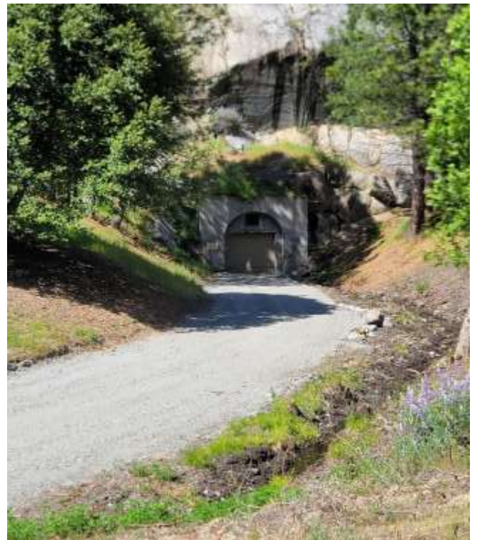
Sandbar Tunnel Access - After
