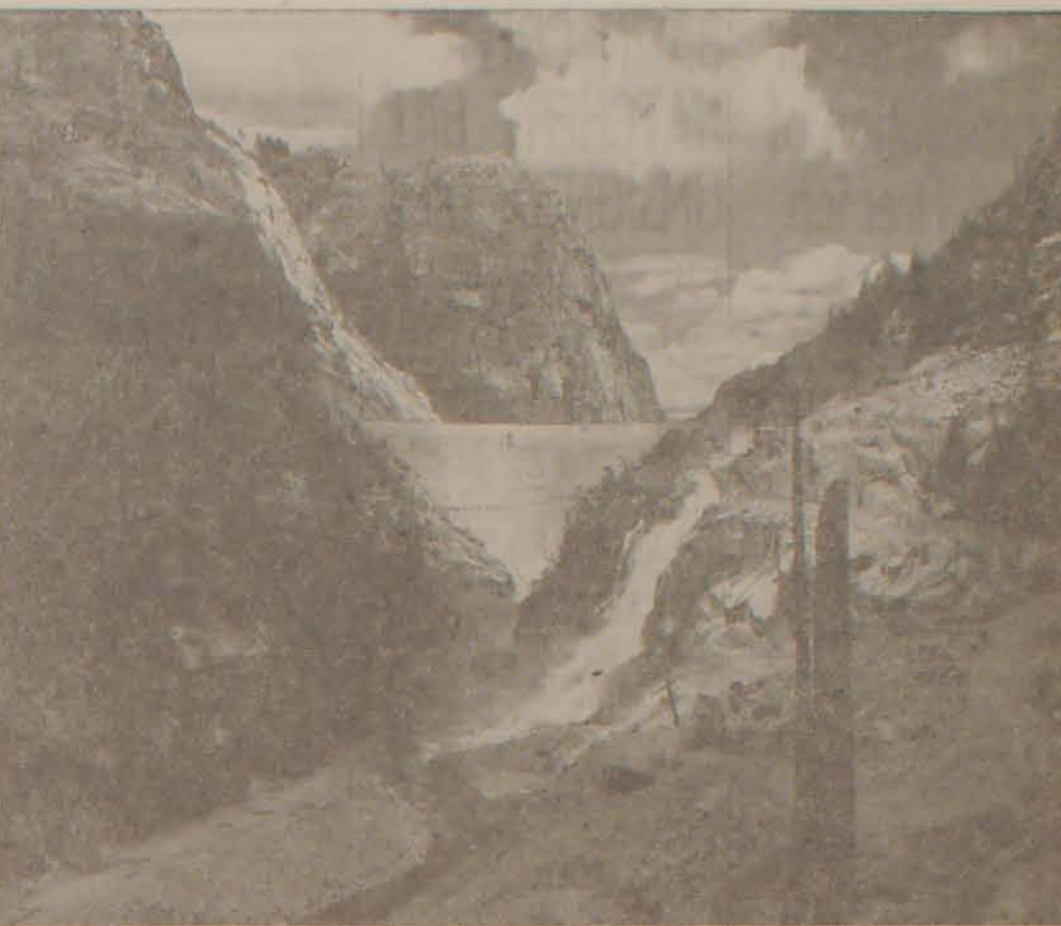
HIGH DAM IS SPILLING —This is a photograph of the completed Donnell's Dam, with water pouring from the spillway at the right. The concrete arch type dam is 10 feet thick at its crest, 290 feet above the stream bed, and 41 feet thick at its base. Water from the reservoir is carried through a seven-mile tunnel, to drop 1,200 feet to the powerhouse several miles downstream.
