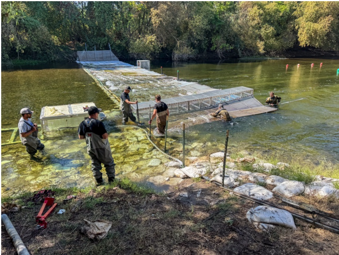
Figure 1. Stanislaus River weir installation.
