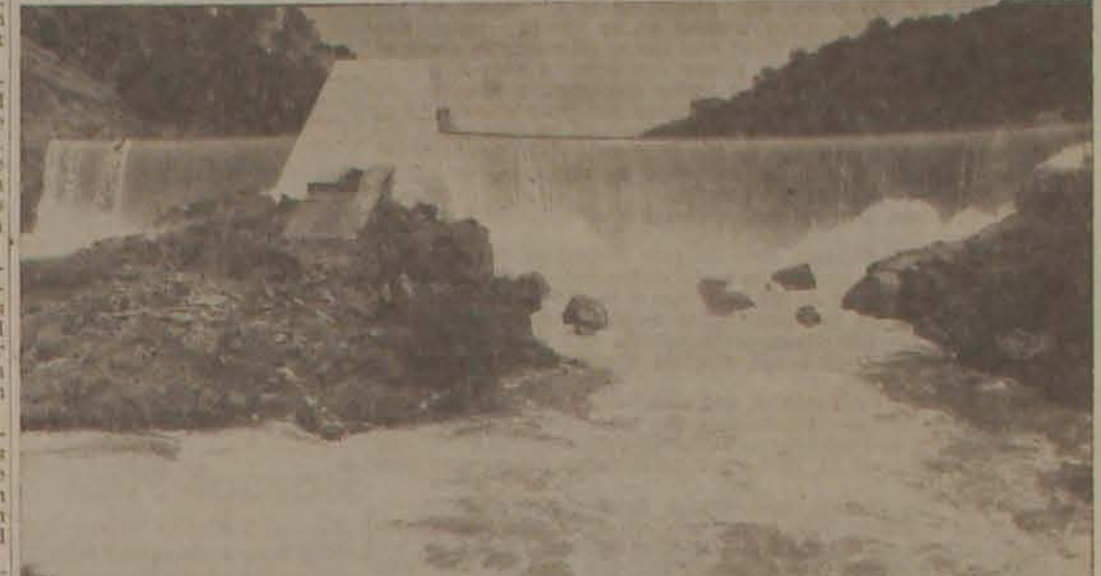
GOODWIN AFTERBAY —This is the old Goodwin Dam after it has been raised seven feet to form an afterbay for Tulloch Dam in order to regulate discharge of water to irrigation district canals. It is known as the diversion works for the irrigation systems.
